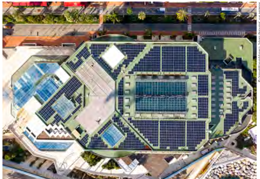
Solar panels on the roof of the Grimaldi Forum
